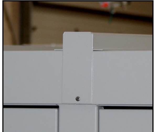
Fig. 11.- Module with covered joint
