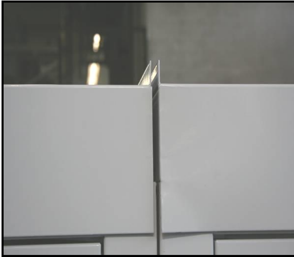
Fig. 10.- Module with exposed joint
